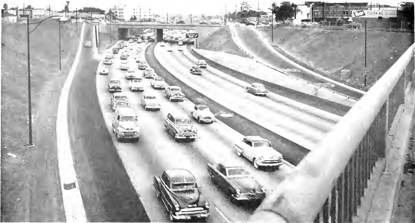
Looking southeasterly along Hollywood Freeway from Wilton Avenue Bridge showing Hollywood Boulevard Overcrossing
